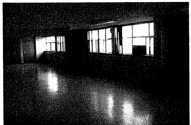
6. View of 3 rd floor meeting room with asbestos containing vinyl floor tiles.
