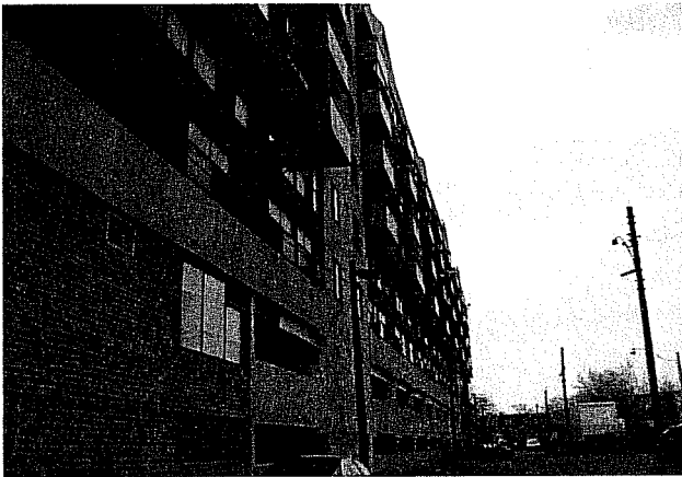
1. Exterior view of subject site facing southwest.
